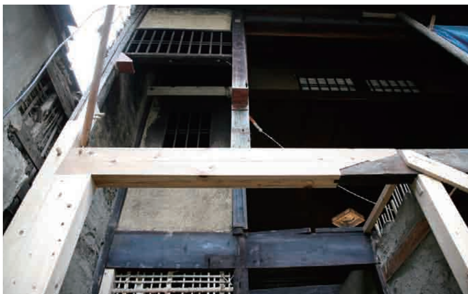
縁側の胴差の腐朽箇所を取り換える repaired beam & support post
