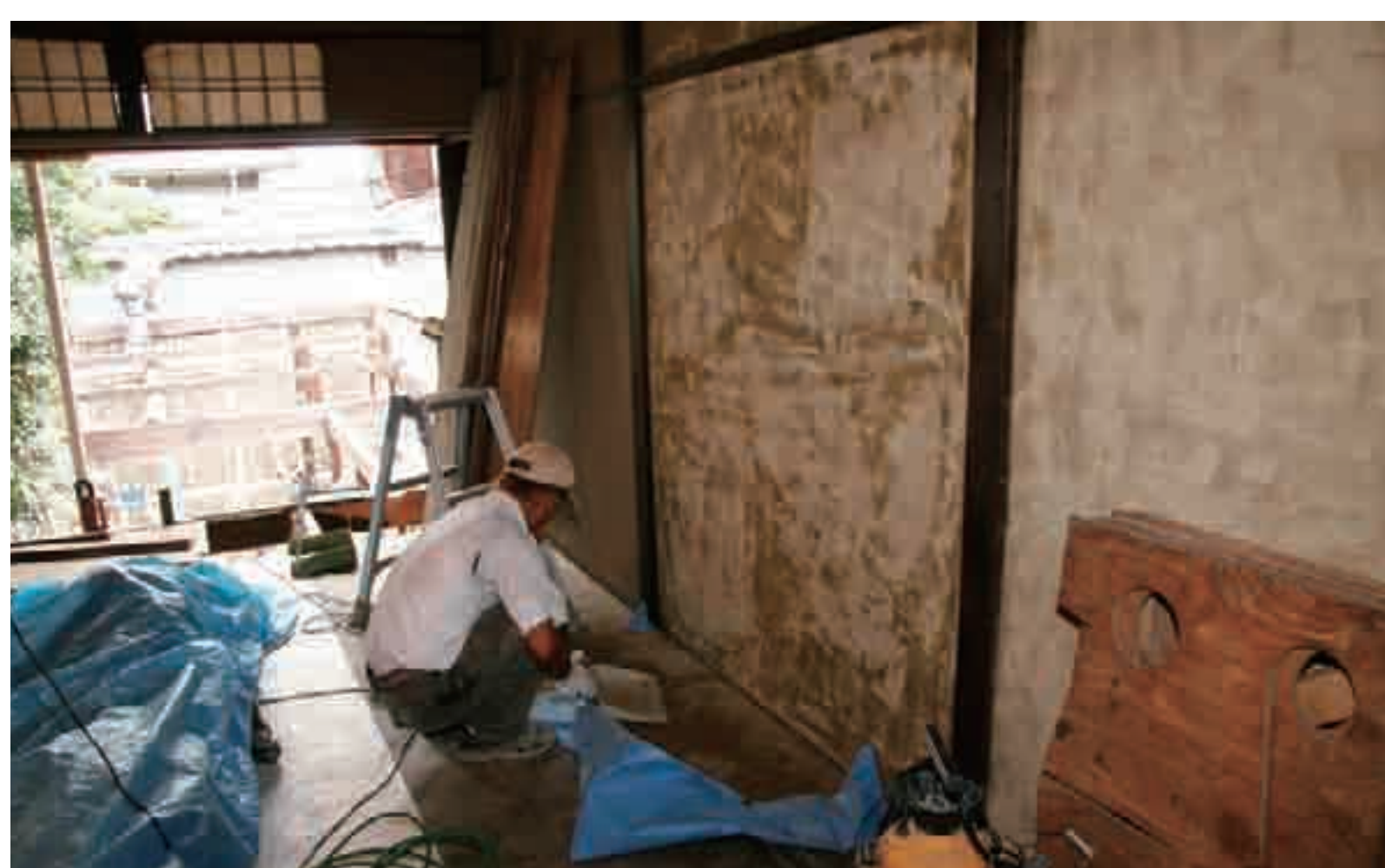
既存土壁仕上層を剥す taking off top coat of clay wall
