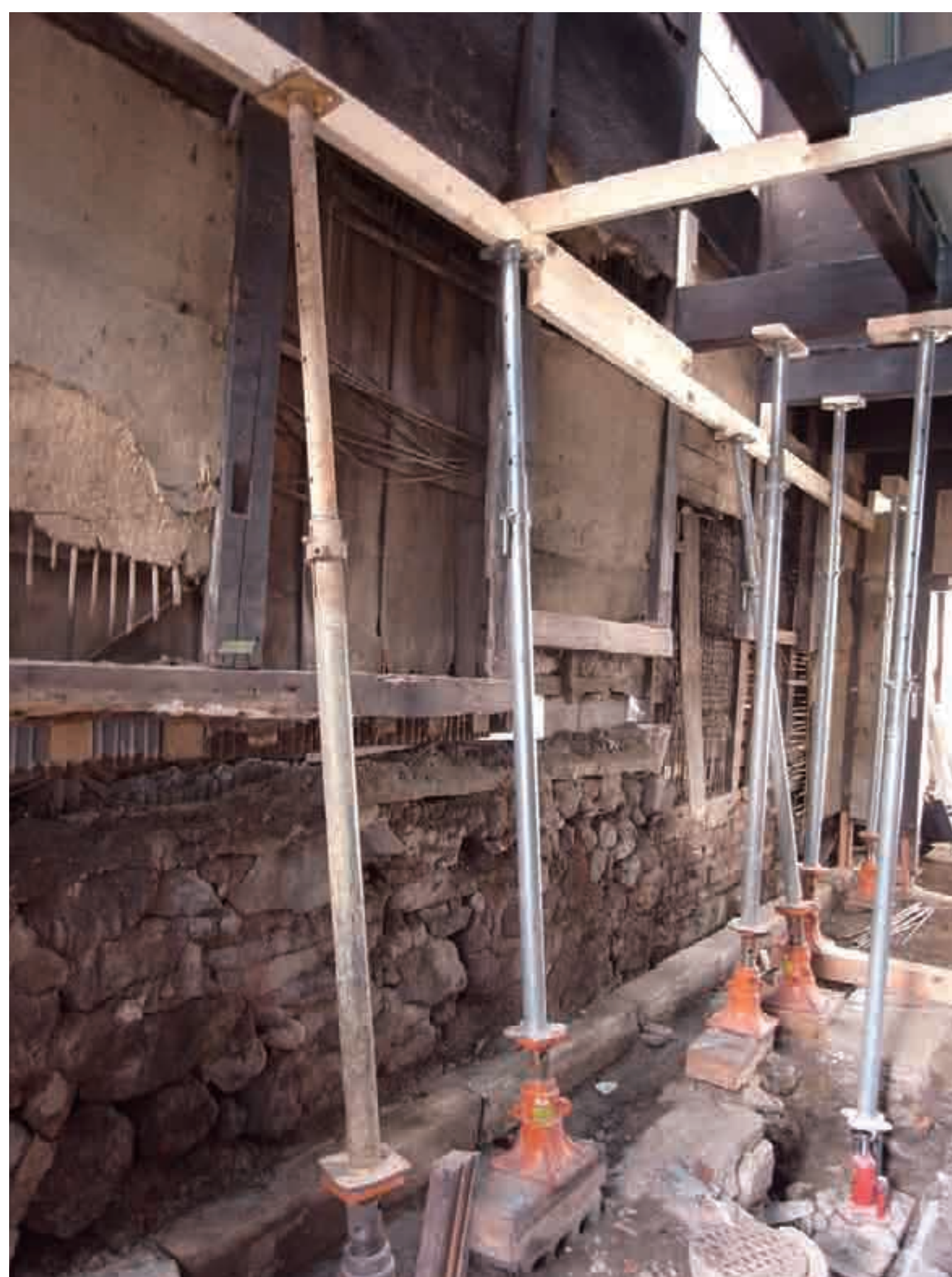
側壁歪み突き retrofitting side wall
