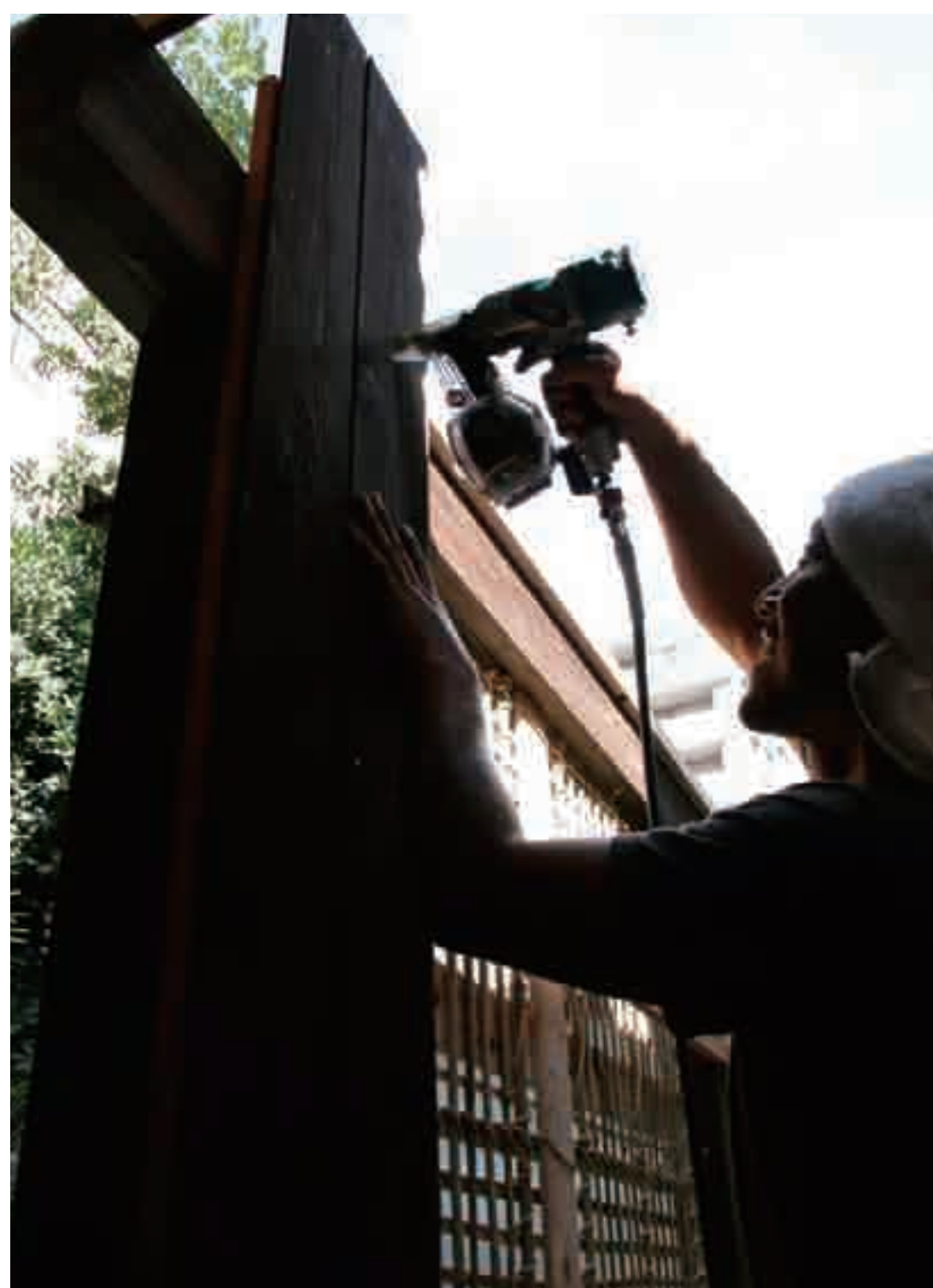
先に竹小舞壁を編み焼杉板を張る weaving bamboo wattle and scorched cedar boards
