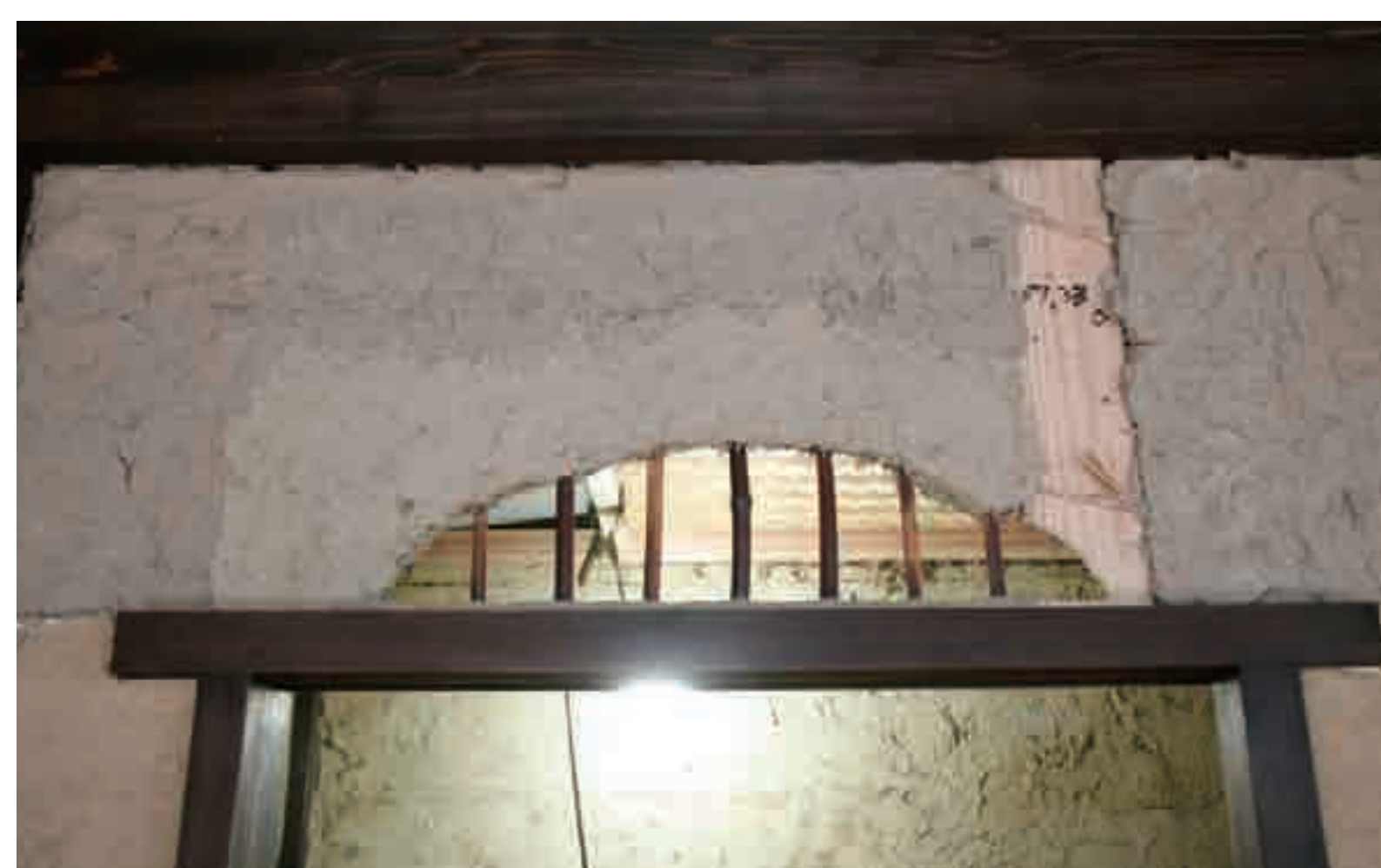
便所入口上部に明り窓を塗り残す substrate window
