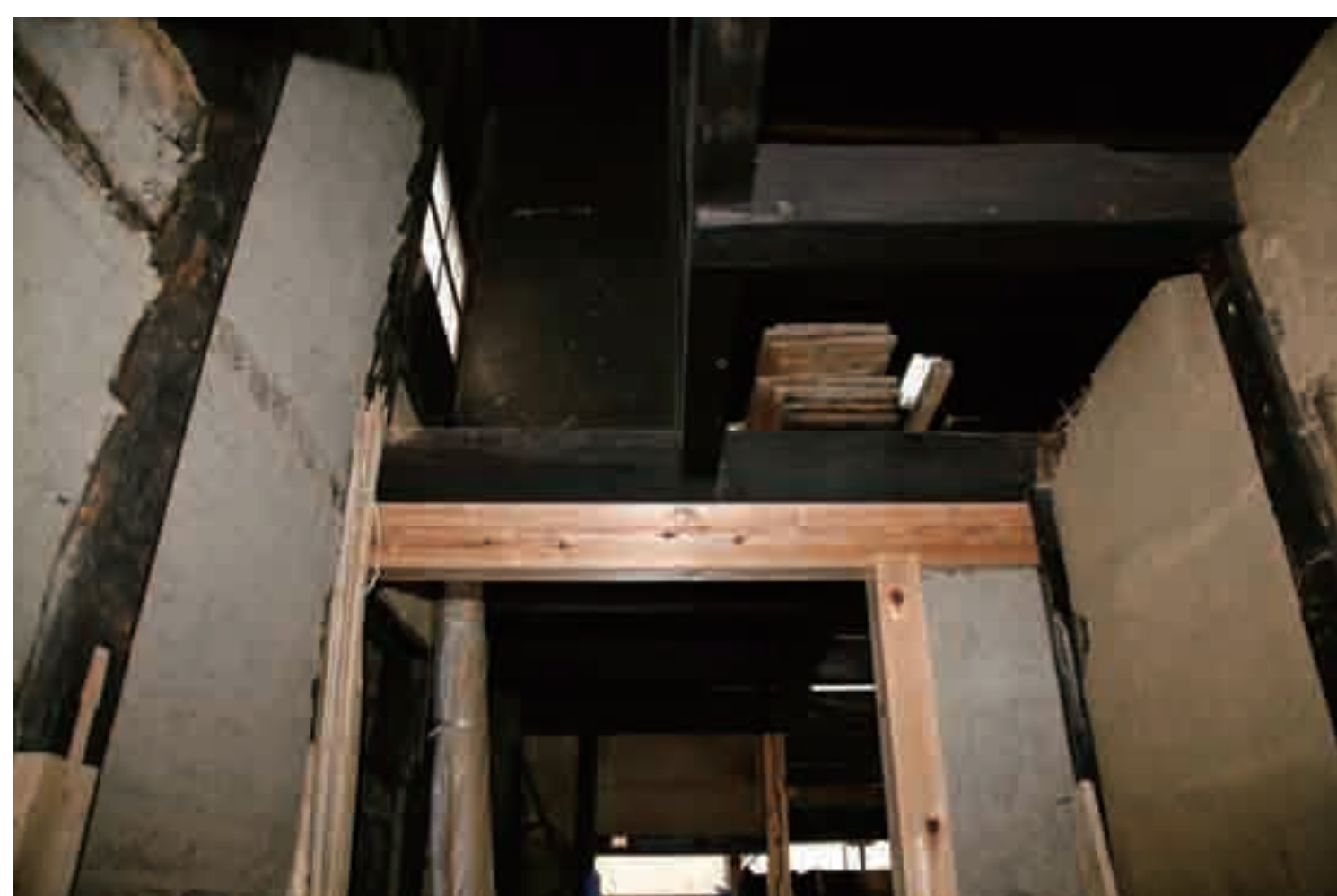
胴差の補強と管柱の差し換え adding support beam & post
