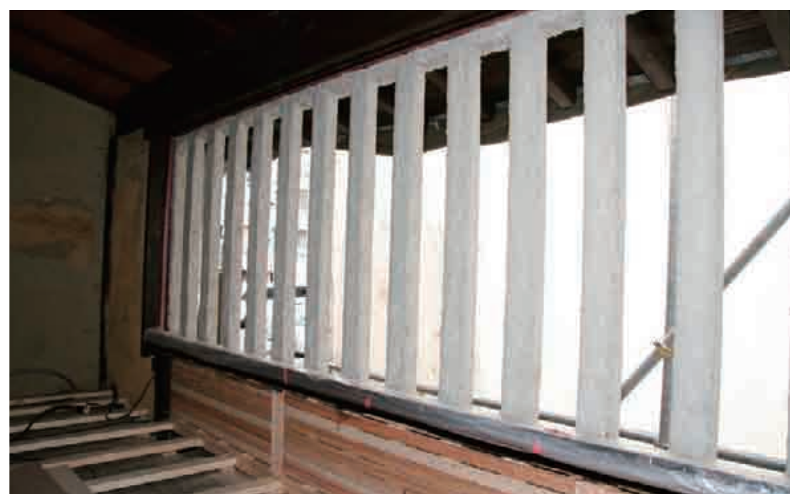
虫籠窓の下塗り substrate plastering of clay lattice window
