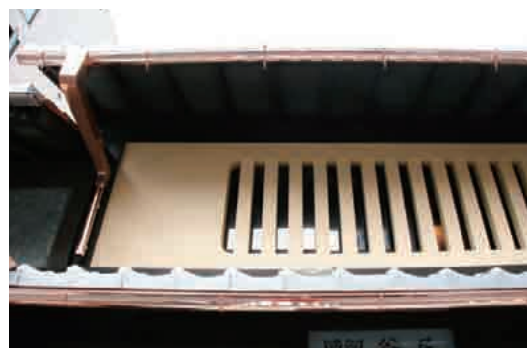
虫籠窓に横樋 clay lattice window & horizontal drain
