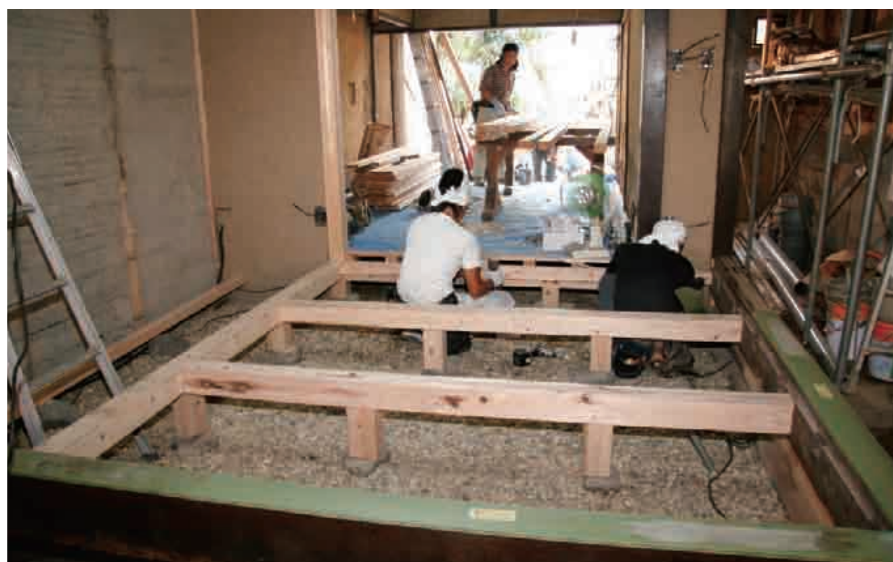
床組 setting new floor structure
