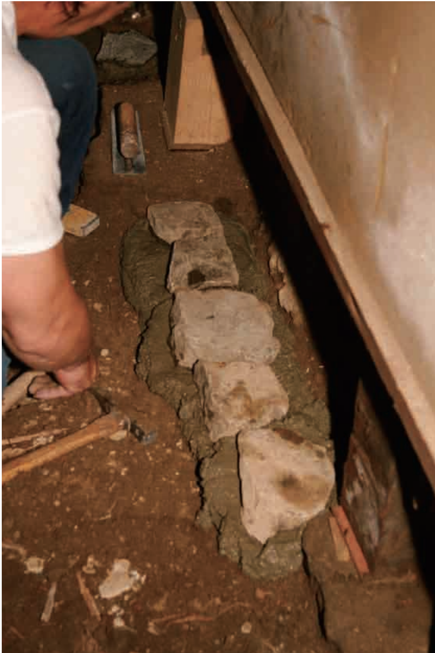
独立礎石を据え直す resetting of individual stones
