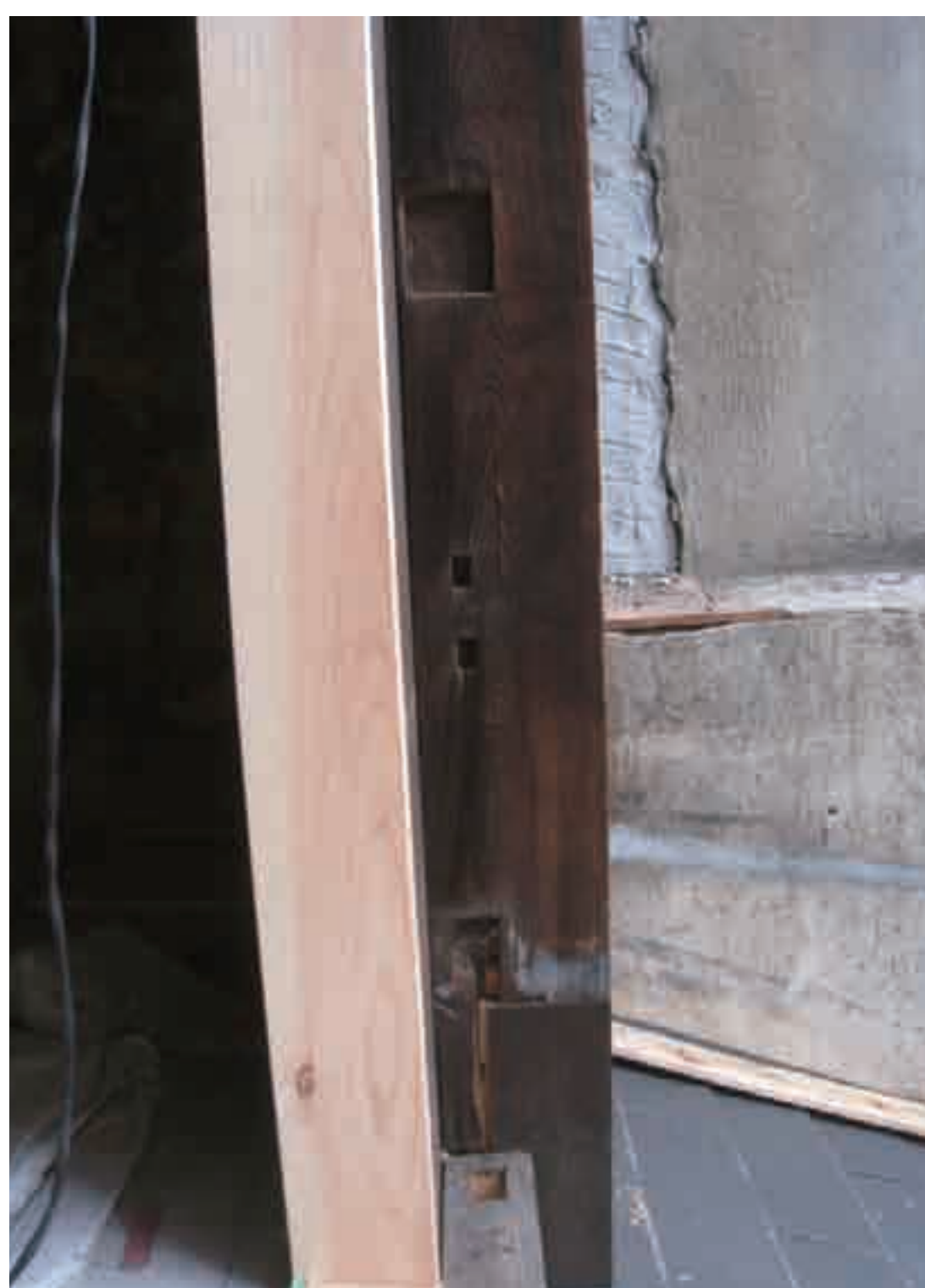
欄干の痕跡 vestigial mortise of exterior railing
